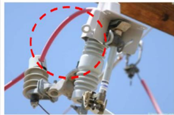
Installation of insulated wires to line facilities to avoid accidental contact.
