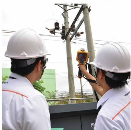
Meralco utilizes its team of experts to provide and maintain the support necessary to ensure that IMI circuit connections are at maximum performance.
