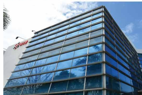
Power-intensive operations at Integrated Microelectronics Inc.'s Biñan, Laguna site requires a proactive energy partner like Meralco.
