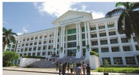
DLSU's Science and Technology Complex in Laguna where Meralco was given a 3,000-square-meter lot for the construction of a substation that will distribute power to the entire campus upon its completion in 2023.
