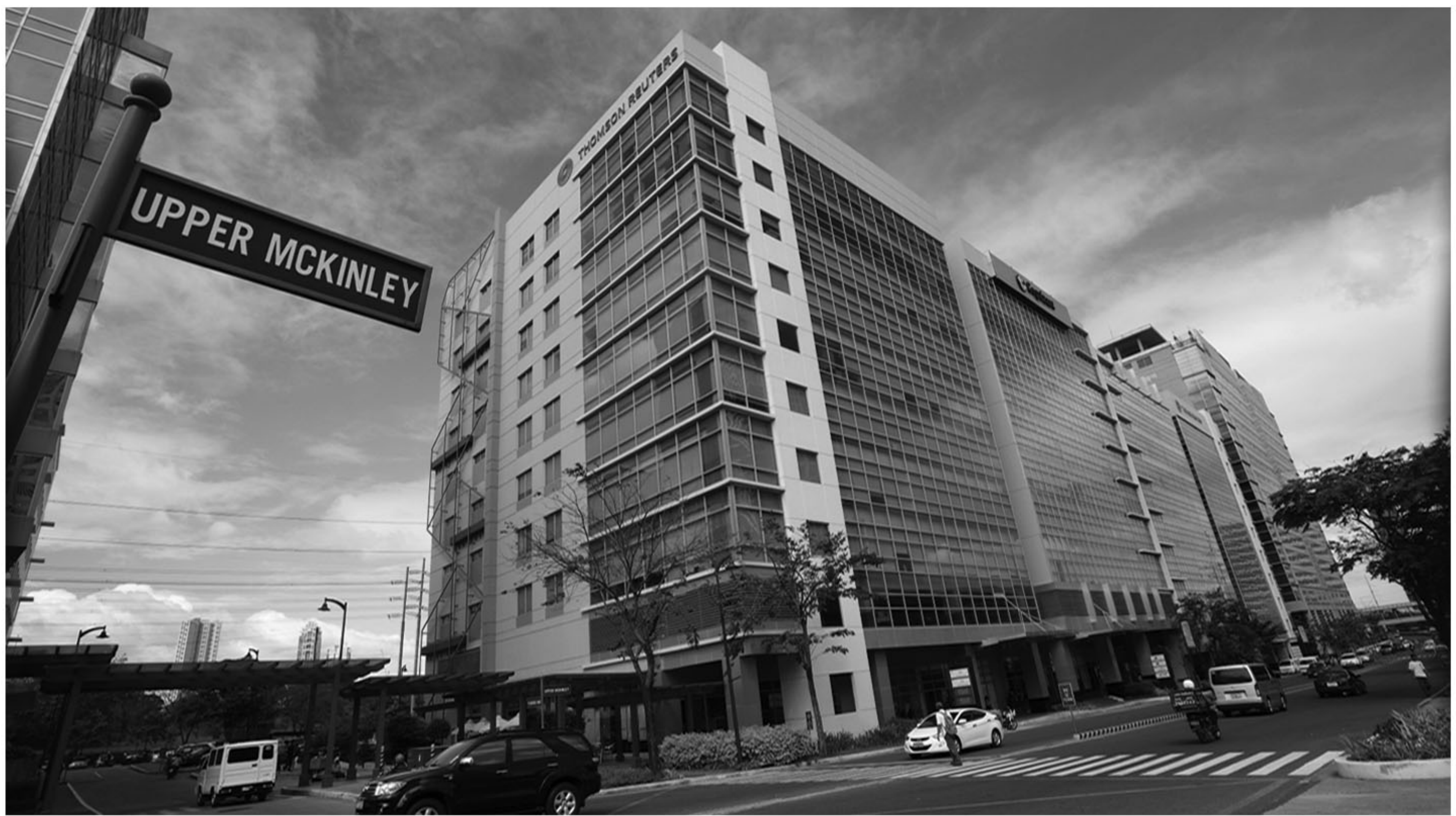
Megaworld's 8 Upper McKinley, one of Manila's premiere KBPO hubs, is an exemplary model of an energy-efficient development which saves its IT-BPM tenants 15% energy costs per month.
