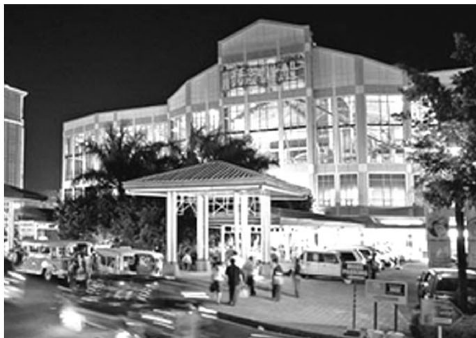
Commercial establishments in Filinvest Alabang are booming with the help of Meralco's Filinvest Substation.
