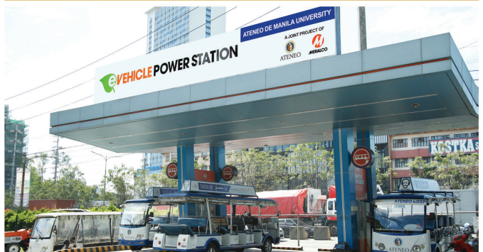
Meralco's subsidiary MServ has been providing operation and maintenance services for Ateneo's six 14-seater e-jeeps and EV charging station since 2009.
